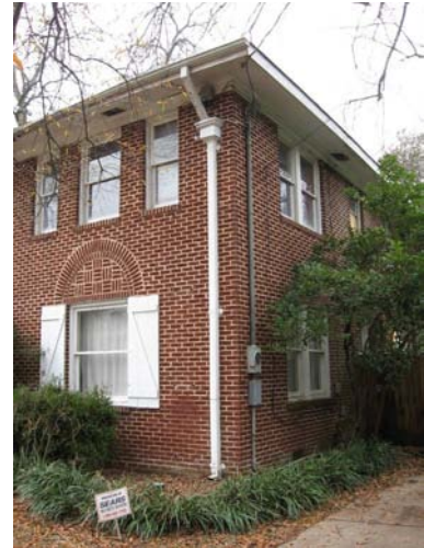
An appropriate gutter and downspout system at 1206 St. John Drive.
