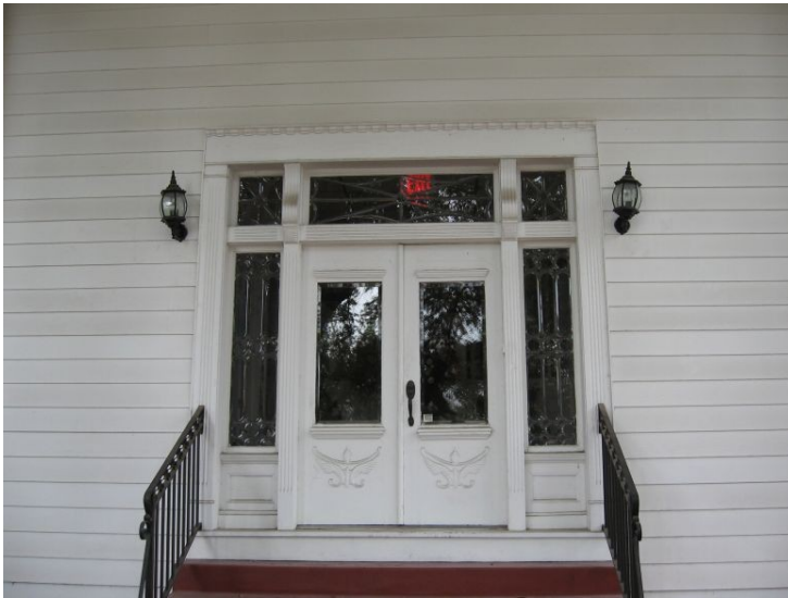
This entrance, with original single-light double doors, sidelights, and transom, convey the historic character of the dwelling.
