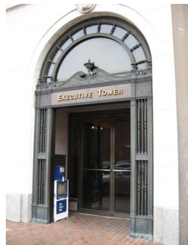
Entrance to Executive Tower at 141 Desiard Street.
