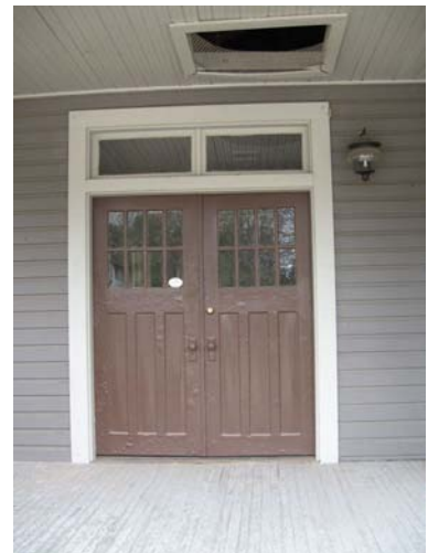
These eight-light, three-panel double doors should be maintained and preserved (1008 N. 3rd Street).
