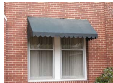
An awning, like this one at 201 Stubbs Avenue, should span the exact length of the opening it is to cover.
