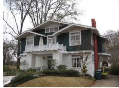
The contrasting colors between upper and lower stories of this Craftsman dwelling further differentiate the wood shingle siding on the top floor from the weatherboard siding on the lower floor (301 Park Avenue).
