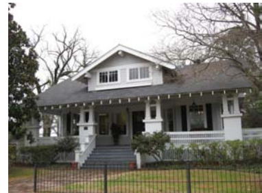
This Bungalow at 903 2nd Street has a full-width porch with paired posts on brick piers.
