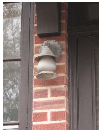
Original light fixture at 409 Auburn Avenue.
