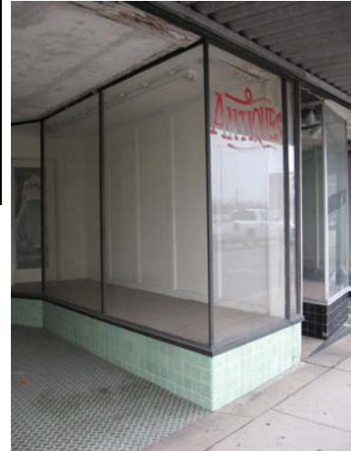
Display window at 408 Desiard Street
