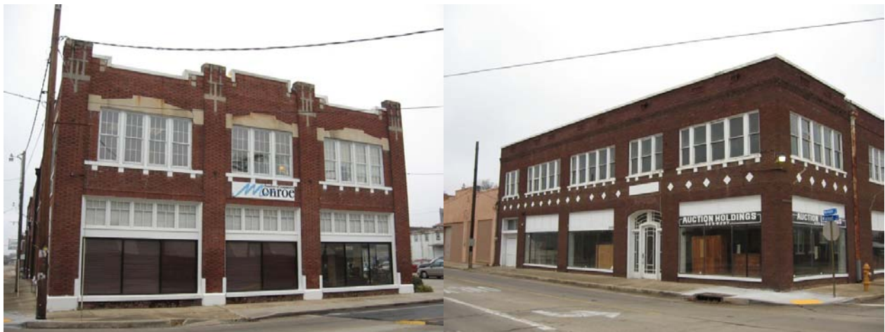
The buildings at 212 (left) and 310 N. Grand Street are examples of Tapestry Brick architecture.
