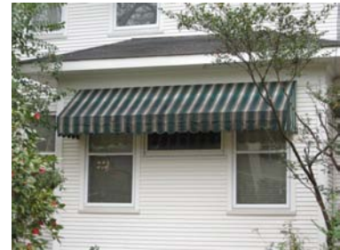
Appropriate awning style and material at 1908 Riverside Drive.
