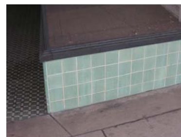
Tile bulkheads such as those at 406 Desiard Street (top) and 408 Desiard Street (bottom) are significant parts of storefronts from the early-to-mid-twentieth century.
