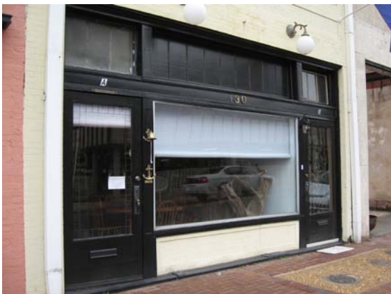
The original storefront at 130 S. Grand Street features single-light glass and wood doors, transoms, and a large central display window.
