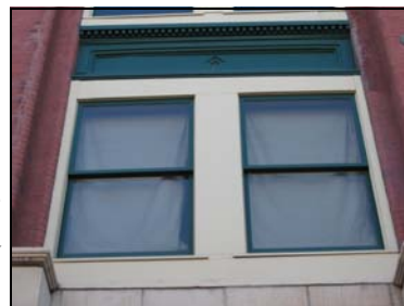
These one-over-one sash windows are a good example of replacement windows. They match the historical design and configuration of the original windows.
