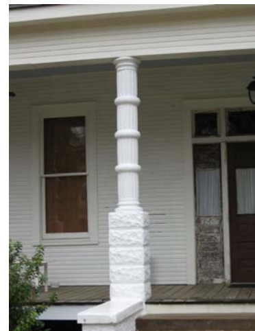
Original concrete porch column at 110 Hilton Avenue.
