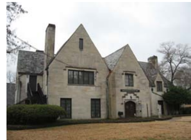
The Masur Museum's steeply-pitched gable roof is a signature of the Tudor Revival style. Altering this roof shape or form would adversely affect its expression of the style.
