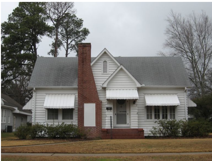
This Tudor Revival dwelling at 201 Auburn Avenue includes the style's characteristic façade chimney, projecting entrance, a cross gable roof, and both wood sash and casement windows.
