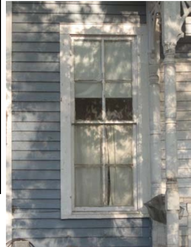
Original four-over-four wood sash windows at 1205 St. John Drive.
