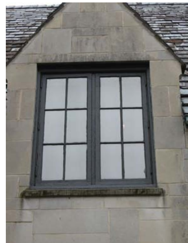
Original casement windows at 1400 S. Grand Street.
