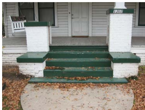
Original concrete steps at 1207 St. John Drive.
