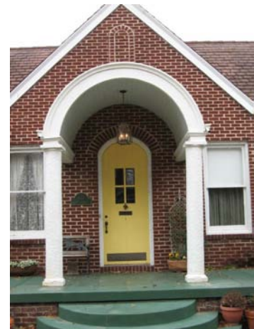
The arched entry porch at 401 Auburn Avenue echoes the arched door and helps define the Tudor Revival style of the dwelling.
