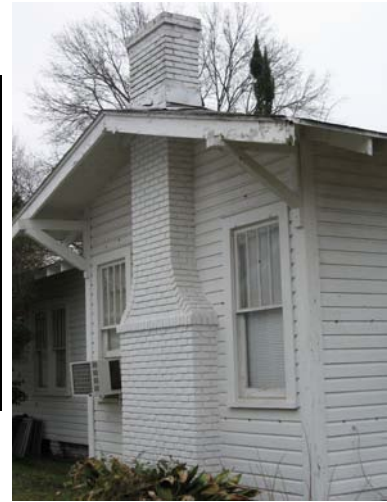
An exterior brick chimney at 1017 St. John Street
