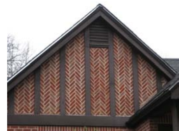
The basketweave brick pattern at 409 Auburn Avenue is a unique feature of the dwelling and should never be painted or concealed.
