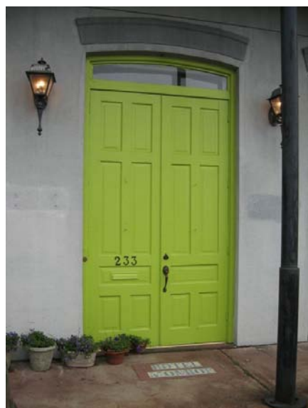
The building at 233 S. Grand Street retains original six-panel doors.
