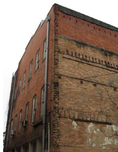
Appropriate rear gutter and downspout at 125 St. John Street.
