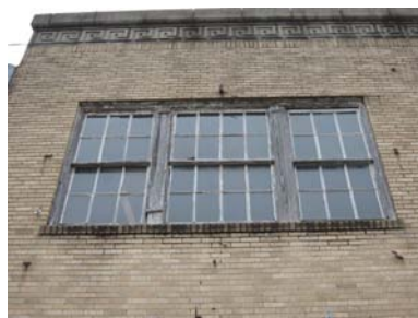
Original six-over-six and eight-over-eight wood windows at 404-408 Desiard Street. This window is significant to the design and character of the building.
