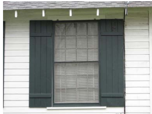
Retain historic shutters like these at 1005 N. 3rd Street.
