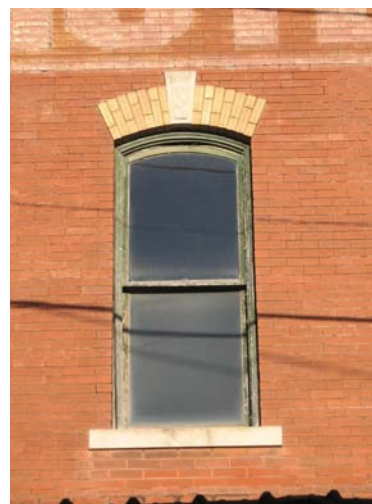
One-over-one arched window with segmental arch above at 500 Desiard Street
