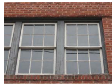
Six-over-six wood sash windows at 117-121 Hall Street.
