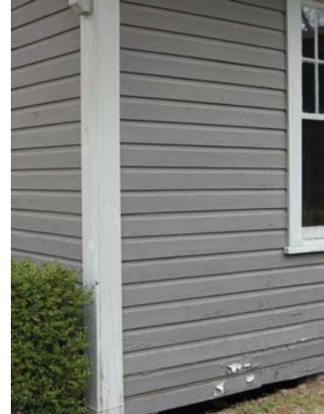
Retain and preserve original wood siding as at 1008 N. 3rd Street.
