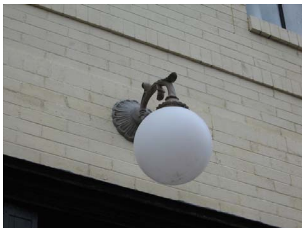
Good reproduction light fixture at 130 S. Grand Street.
