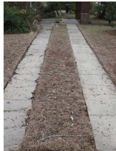
The "ribbon" driveway design is a common historic design (400 Auburn Avenue).
